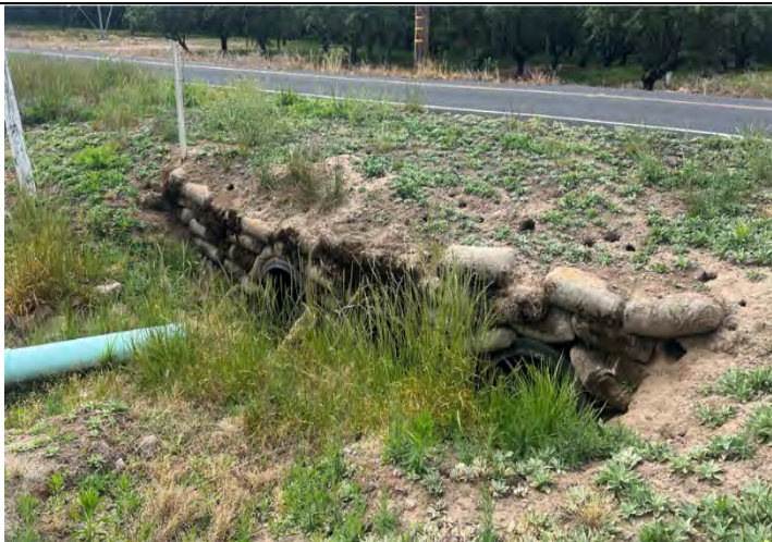
Photo 21: Location of proposed Sand Creek Culvert #2, facing south.
