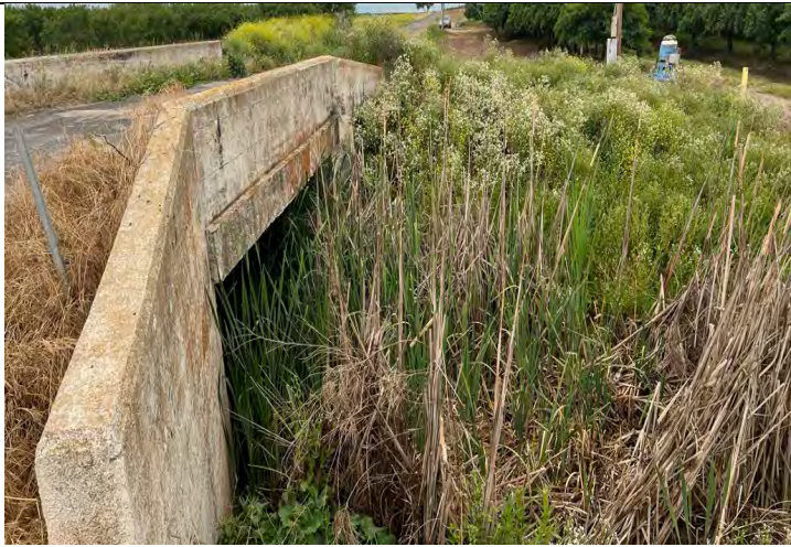
Photo 25: Mustang Creek (MC-1) Culvert, adjacent to E Monte Vista Ave. Facing east.
