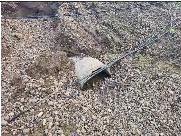
Photo 12: Representative photo of a culvert at DP4 facing southeast.
