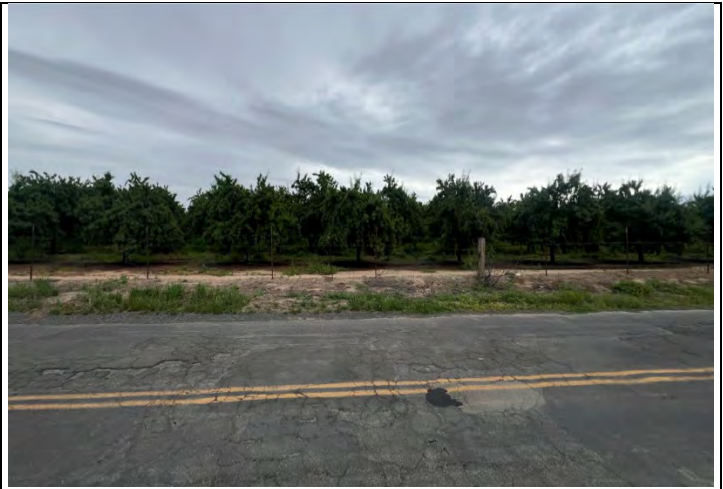
Photo 20: Location of proposed Sand Creek Culvert #1, facing east.
