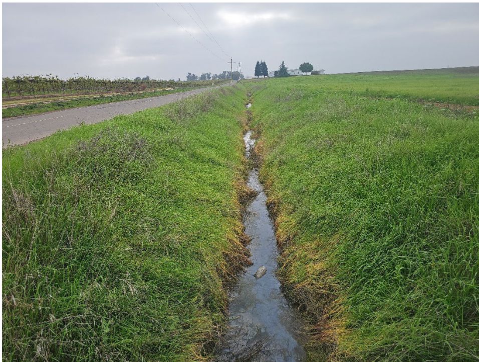
Photo 6. View of the ephemeral drainage that intersects Mustang Creek. View facing west.
