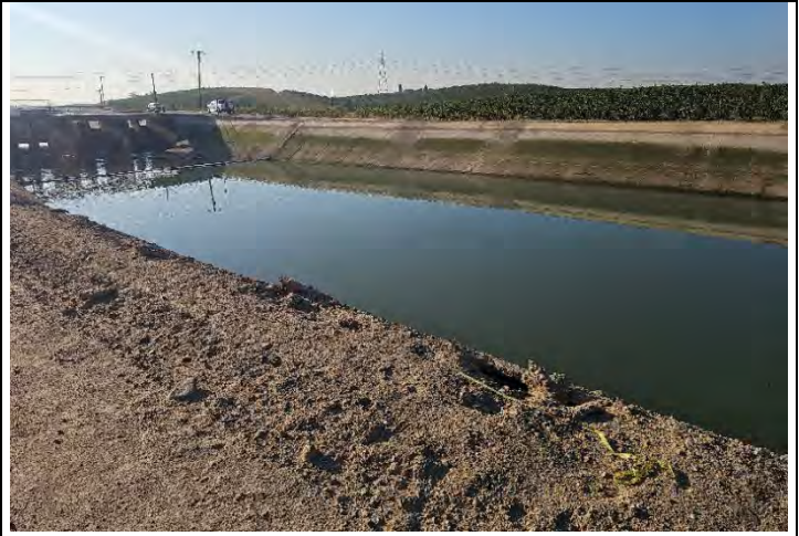
Photo 14: Turlock Irrigation District Main Canal AW-1, representative photo northeast.
