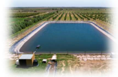
Recharge / Retention Ponds
